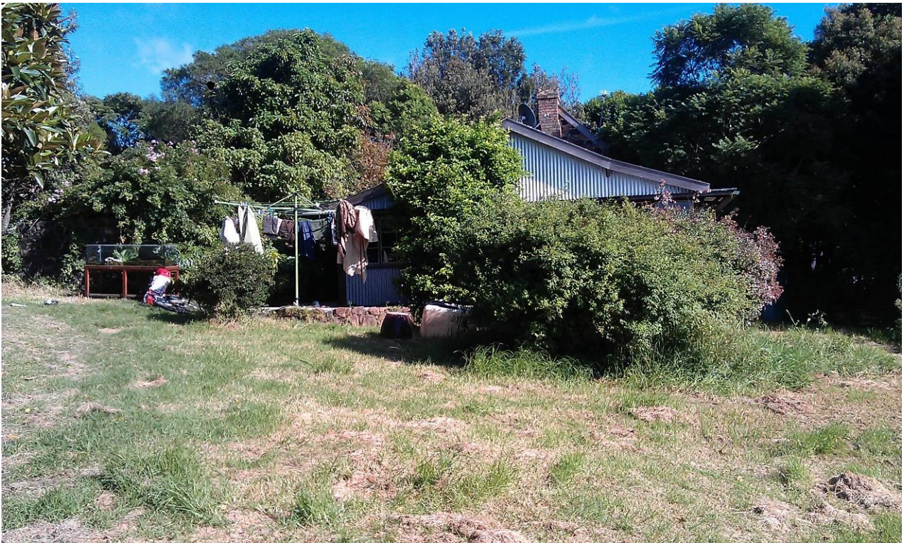
Figure 5 – View west over cottage. Septic tank in shrubs in foreground.
